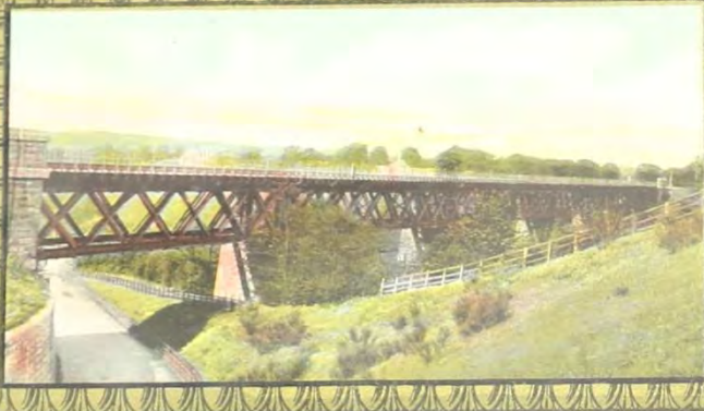
THE VIADUCT, LARKHALL.
