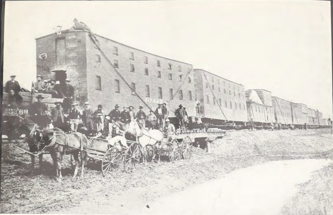
Construction crews on the St. Paul, Minneapolis & Manitoba—the Great Northern's predecessor—took their own out-size dormitory cars with them as they pushed the road across North Dakota and Montana late in the 1880's. Farther west, the cars had to be sawed down to get through tunnels dug in the mountains. Soldiers went along to ward off hostile Indians.
